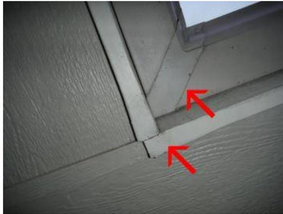
Evidence of leaking is noted at the gutter joints. This can cause damage to fascia. Recommend re-sealing joints and end caps.
