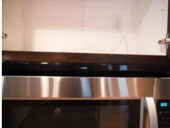
*The microwave as installed is recirculating back into the home even though there is a vent line running through the roof. Recommend turning the fan on the microwave to vent properly outside.*
