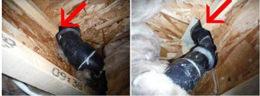
*Floor joist was cut under the hall bathroom toilet and the shower to fit plumbing line through without adding additional support. Recommend installing support under floor joist.*
