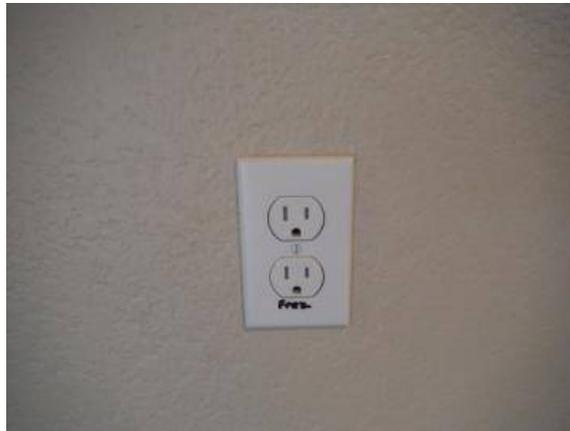
*One outlet in the garage labeled freezer is not properly GFCI protected as needed. In 2010 dedicated outlets were not permitted and even when they were dedicated outlets has to be a 20 outlet and circuit. This one is a 15 amp. Repairs needed.*
