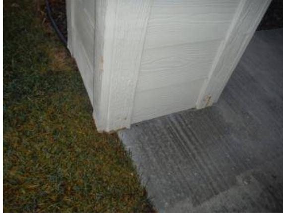
Evidence of sprinklers spraying on the back patio posts, this can cause damage. Recommend adjusting or moving sprinklers to not spray on the siding.
