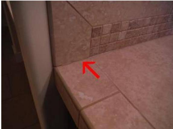
Caulking is needed along the counters in the bathroom.
