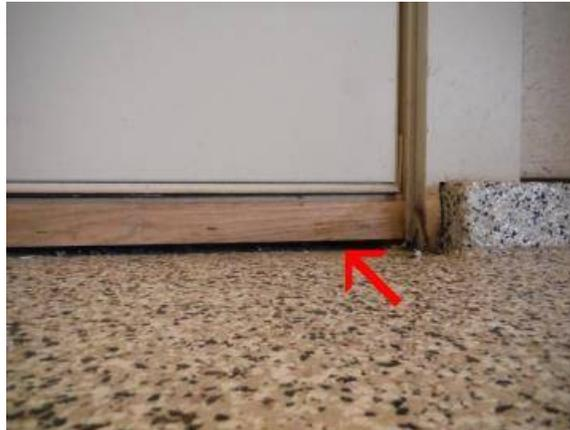
Gap is visible under the threshold on the outside entry door to the garage, with evidence of past water entry. Recommend sealing.
