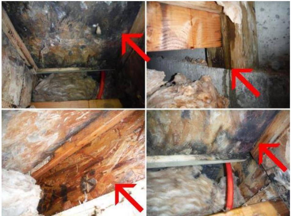
*It appears the shower pan is leaking into the crawl space. Water is dripping out from around the shower area in several places and moisture is noted under the tile with a moisture meter. Damage to the sub-flooring and microbial contamination from the leaking is visible under the shower area in the crawl space. Recommend further evaluation and repairs as needed by a professional contractor for likely replacement of the shower area.*
