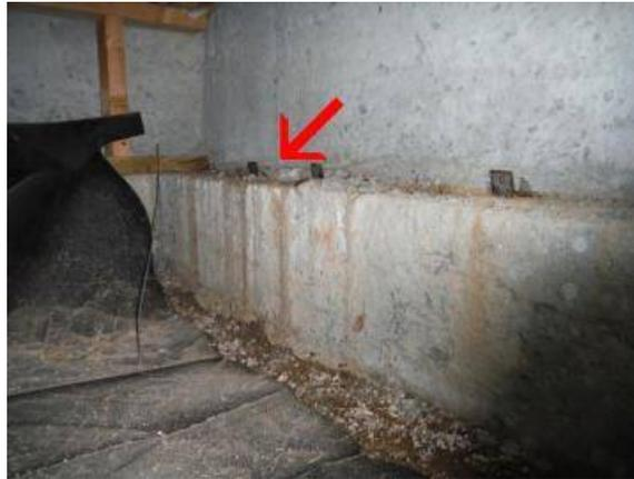
Evidence of past water entry is noted in to the crawl space, Ground should slope away from home. Extend gutters away from foundation. Adjust or move sprinklers away from the foundation.
