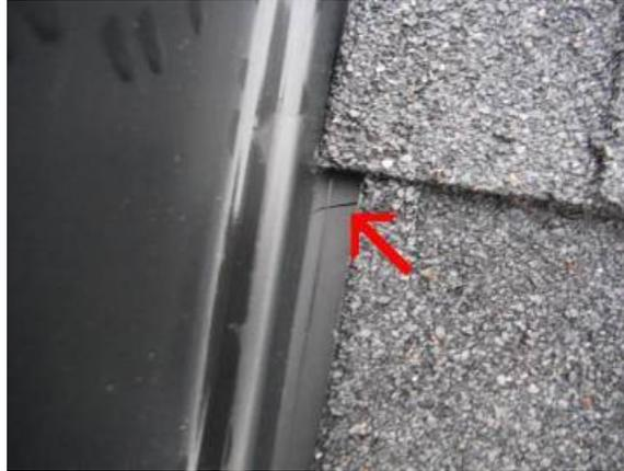
*Small crack is visible in the dryer vent cover on the roof, recommend sealing or replacing.*
