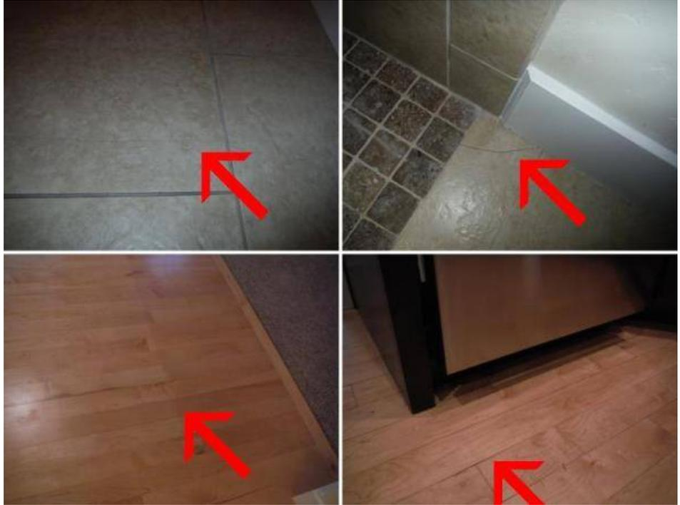
*Couple of tiles are cracked at the entry to the master bathroom and one by the shower in the NE bathroom.*
