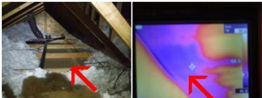
*Insulation over the NE bathroom has been moved for some repairs and not replaced. This is visible in the attic and with a thermal camera, recommend repairs and adding additional insulation if needed.*
