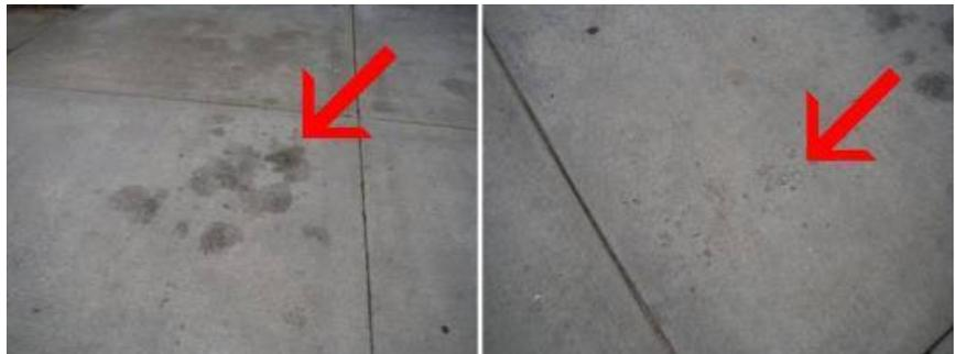
Spauling is noted on the driveway. This is typically from over salting, although it is not a fatal condition it may continue to deteriorate.
